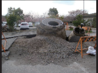
Sand blow, floating of buried objects and sinking of roads due to liquefaction
