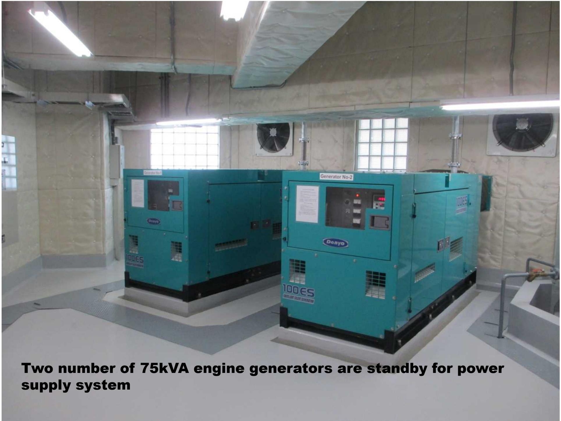
**Two number of 75kVA engine generators are standby for power supply system**
