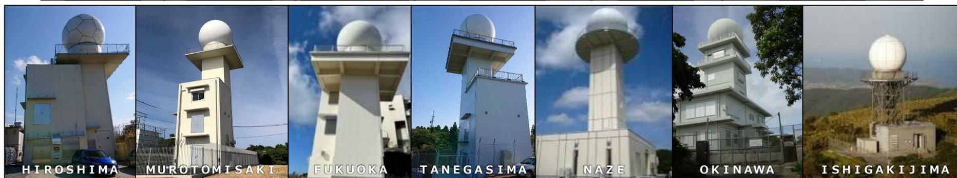
Sites are chosen with focus on high-altitude environments and elevated antennas to prevent radio-wave blocking. They are free-standing and uninhabited, except those at the radar-managing local offices in Akita, Sendai and Nagoya.
