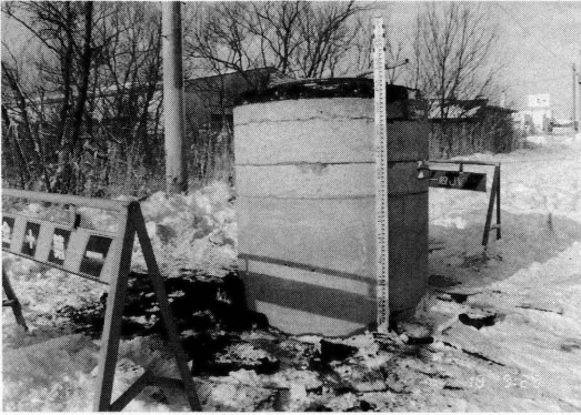
Fig. 2.5 This manhole was raised from underground due to liquefaction. (Kushiro-cho, Kushiro-Shicho)
