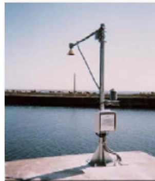
◆ Acoustic Type Gauge Station
