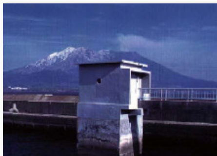
◆ Stilling-well Type Gauge Station
